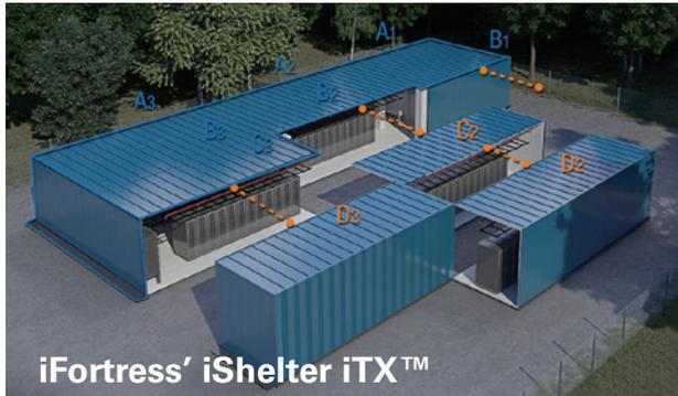
The iShelter iTX™ is designed for exterior or brownfield locations. It is pre-configured at an off-site facility and shipped in a series of interlocking decks to be sequentially linked to create a singular assembly at the designated site.
